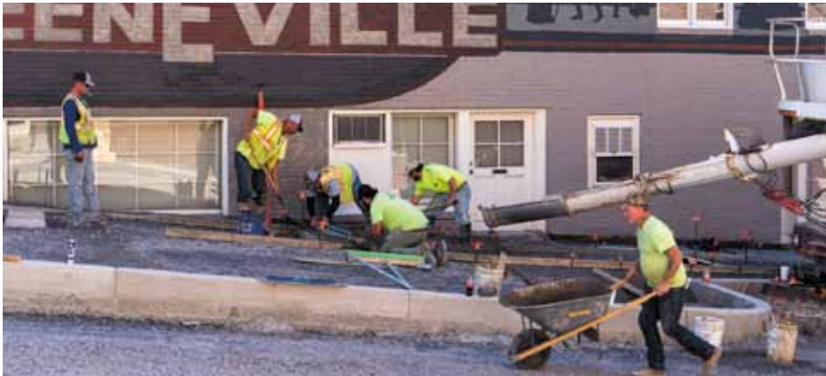
Construction teams from Summers-Taylor are busy pouring sidewalks along Depot Street.
